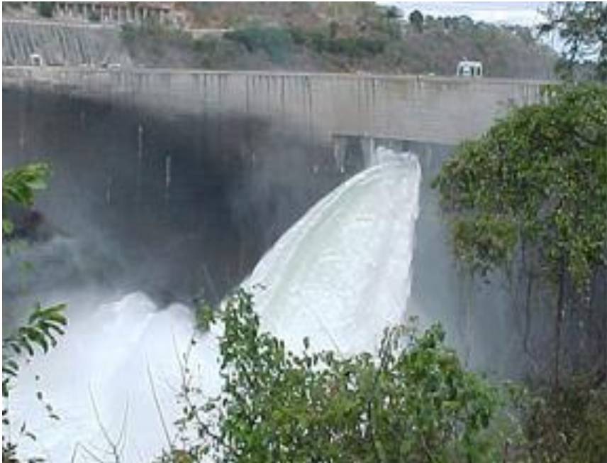
Kariba North bank power supply
