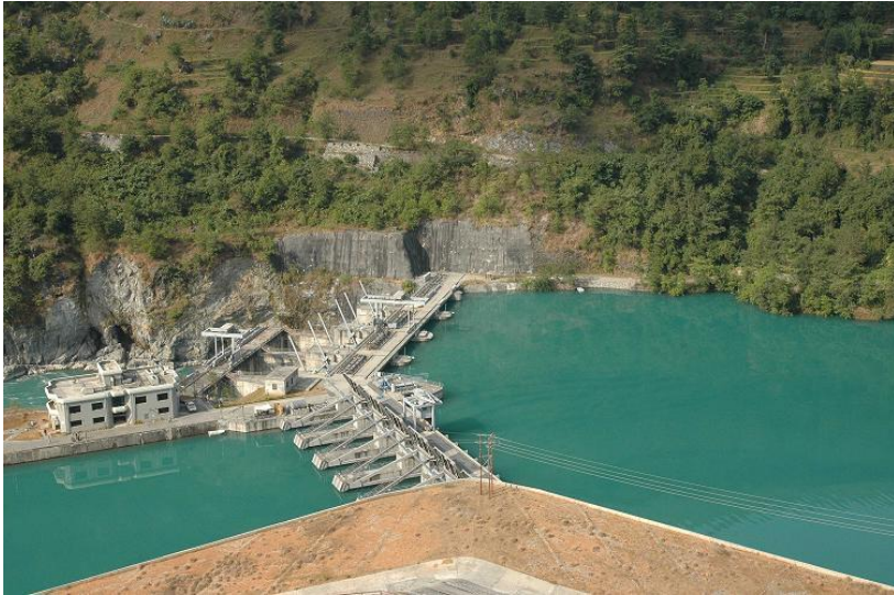
Kali Gandaki Hydropower
